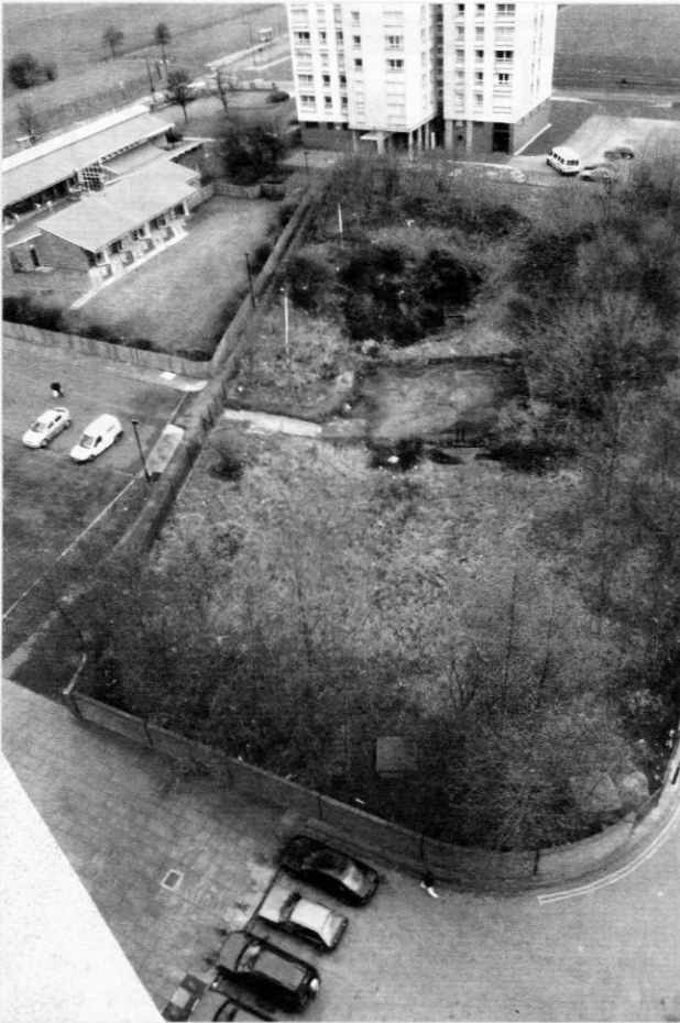
The site of the Group Control filter room at Blakelaw seen from the roof of an adjacent block of flats.
